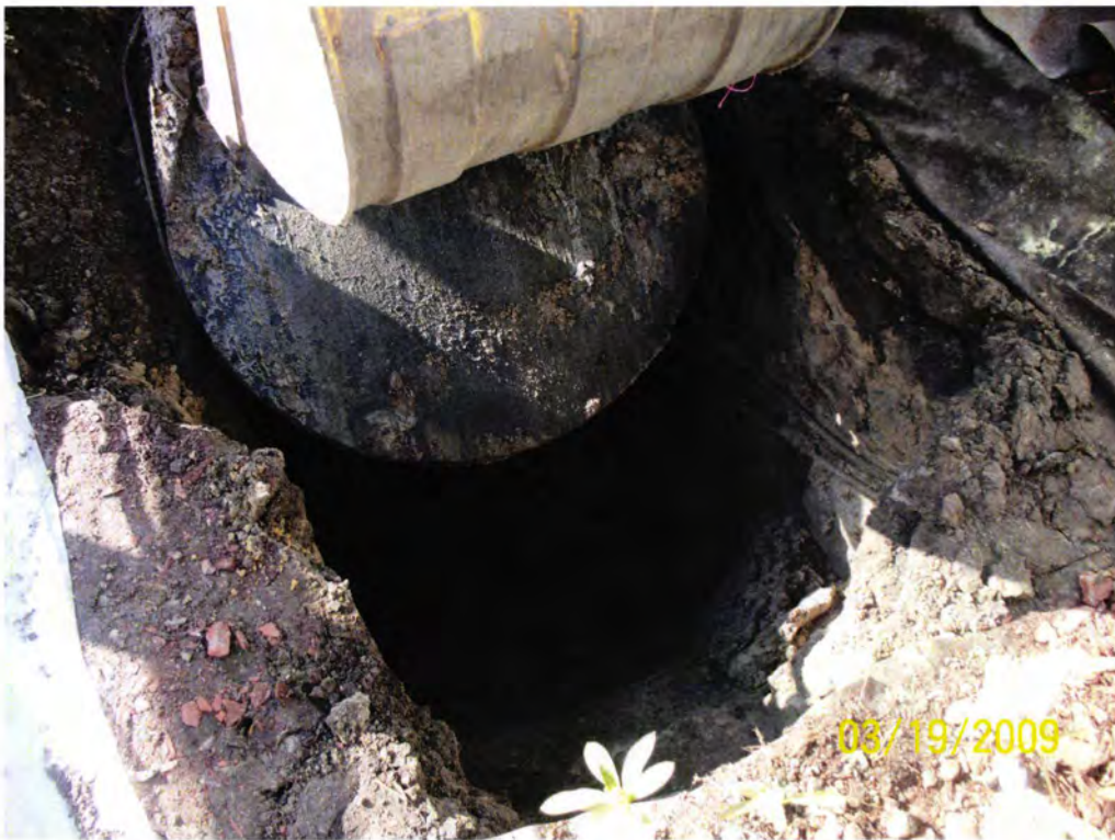
Picture 2: UST 148 Laurel Bay Blvd being removed from the excavation.
